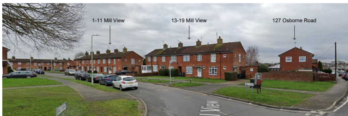
Figure 4 - Previous dwellings (now demolished)
